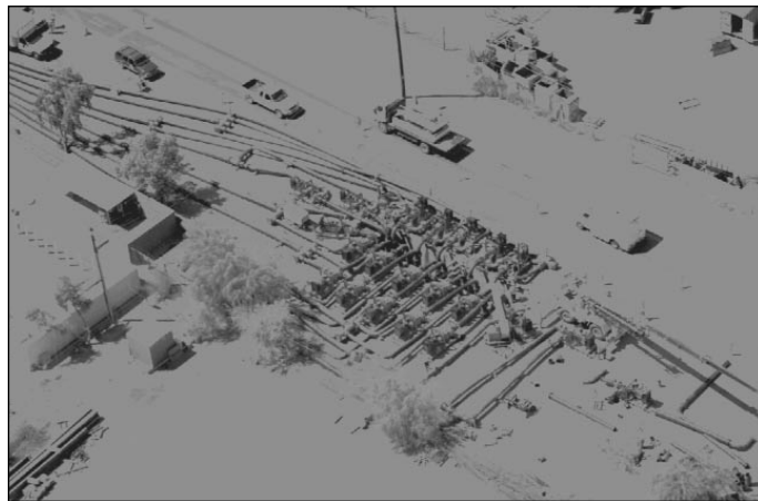
150-mgd Bypass Operation During Pipeline Rehabilitation
