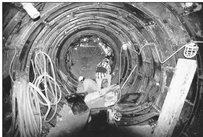
Linear Plate Tunnel
