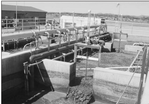
Plant in operation seeded with 20,000 gallons mixed liquor
